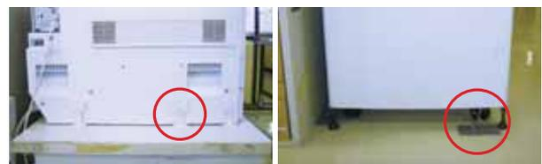
Color printer is now anchored to base plate.
